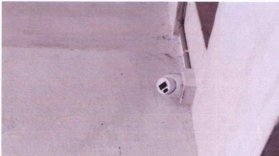
Camera placed in the corridor
